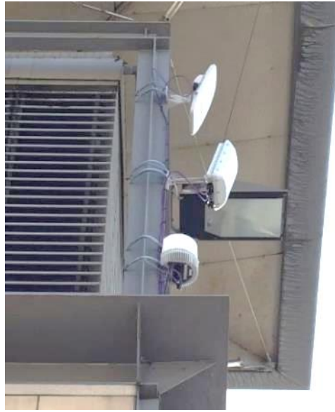
Figure 66: Wi-Fi APs in Millennium Square
