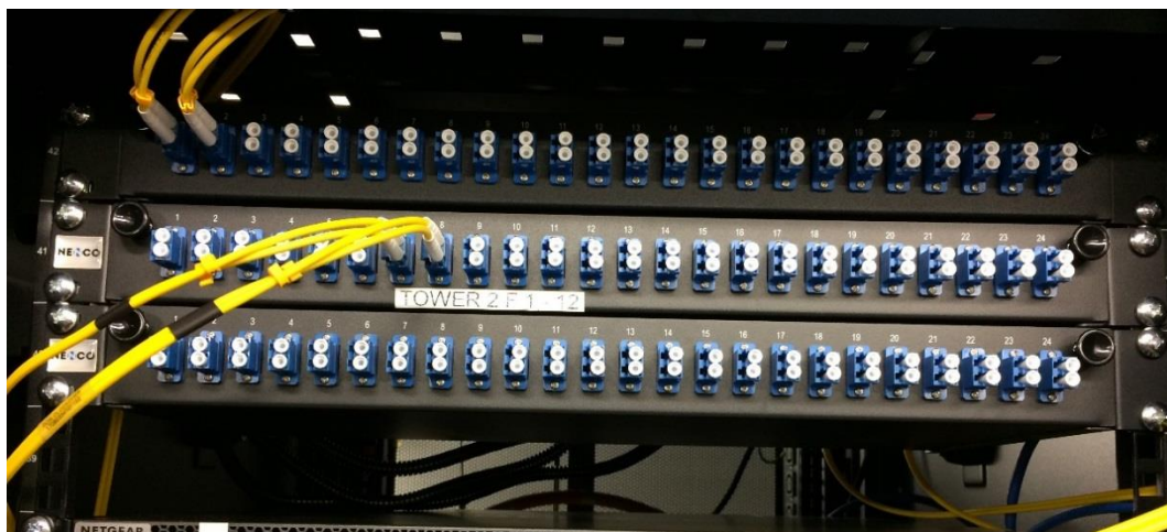
Figure 72: Termination of single optical spoke in distribution node
